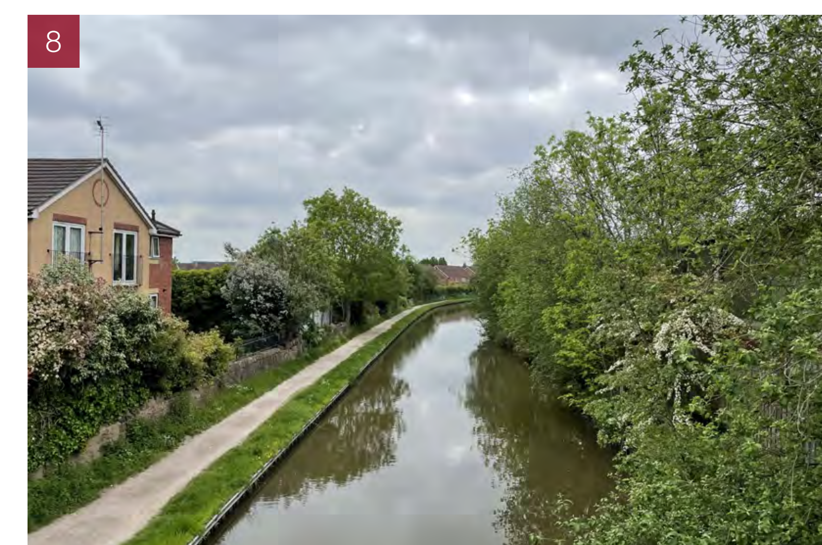
Bridge over the Coventry Canal
