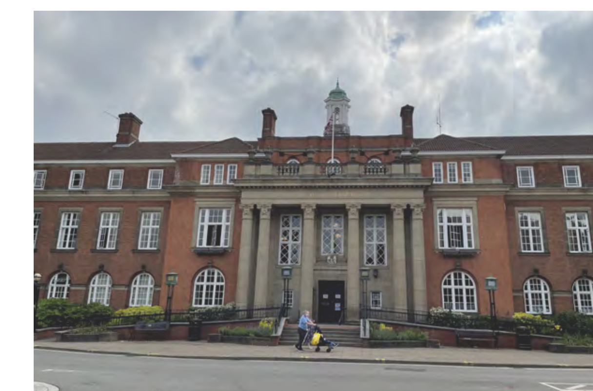
Nuneaton Town Hall
