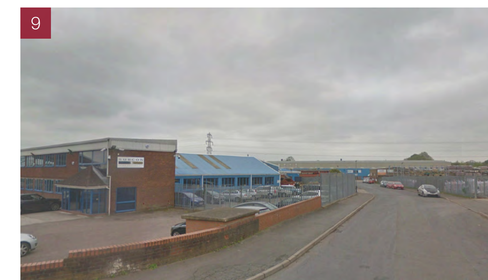
View looking west along Hazell Way
